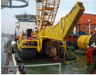
Sister Trencher with Chain Cutter and Jet Pumps offshore Holland
