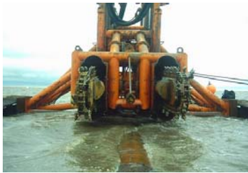
Pipeline Sister Trencher Performing Shore Crossing in Russia in Summer
